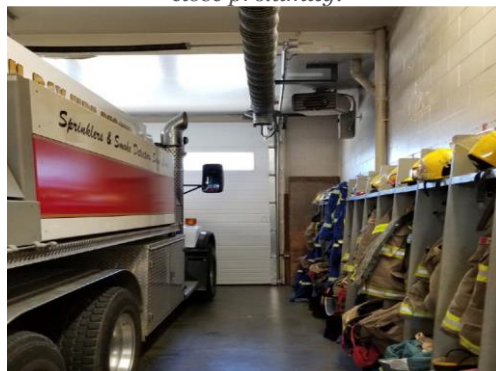
Figure 3: Views showing the small apparatus bays that force vehicles to be parked closely together with turnout gear change areas in close proximity.
